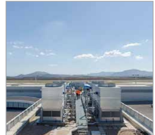
Athens International Airport, Supply & installation of Water-cooled chillers
